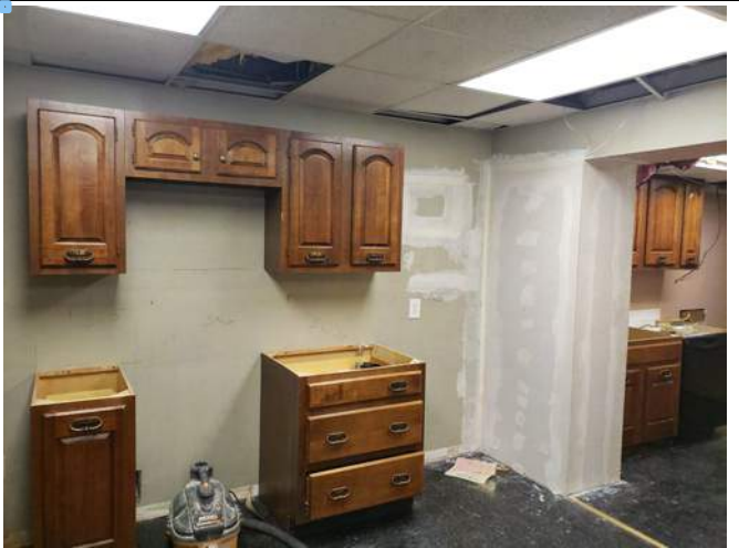
Building a new kitchen in the basement
