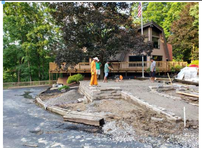
Filling and tamping limestone
