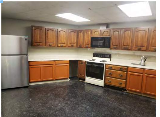
Completed new kitchen
