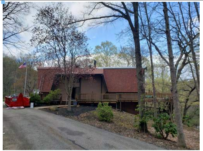
Building with new colorful shingles
