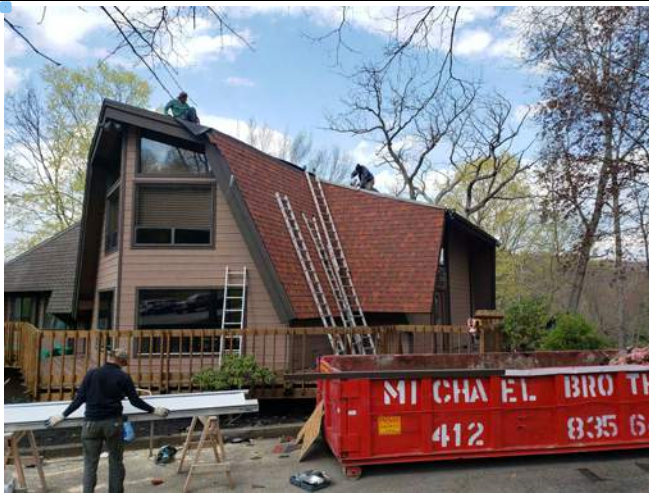
Laying new shingles
