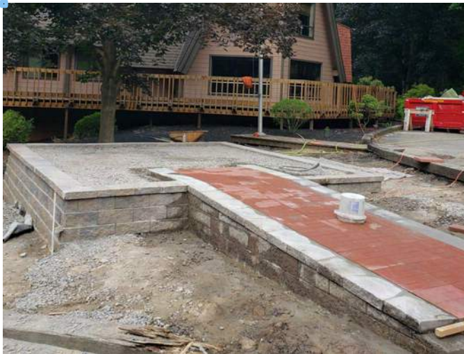
Platform completed with Ven. Metta's direction
