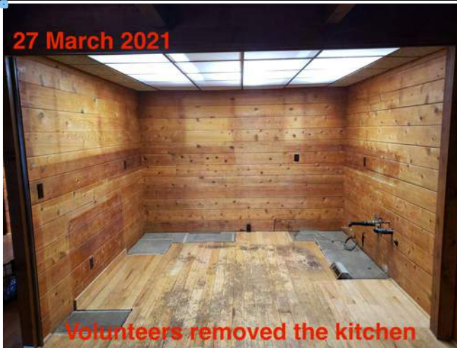
Removing the old kitchen floor
