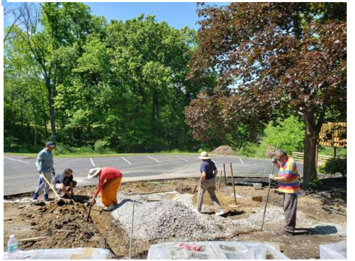
Breaking ground for the statue platform
