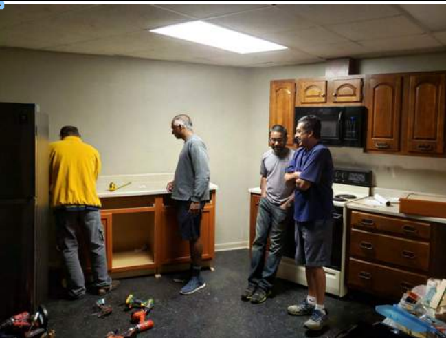
Volunteers assisting to build the kitchen
